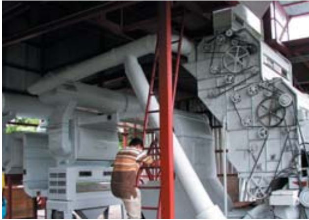
Jubilee House purchased a used cotton gin from El Salvador and set it up next to the spin plant construction. Photo: JHC-CDCA
