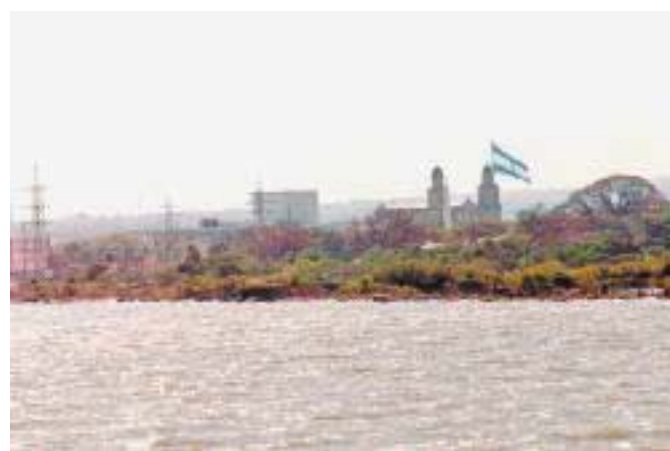
On Feb. 20, ENACAL inaugurated a new sewage plant for Managua that will help clean up Lake Cocibolca. Photo: La Prensa
