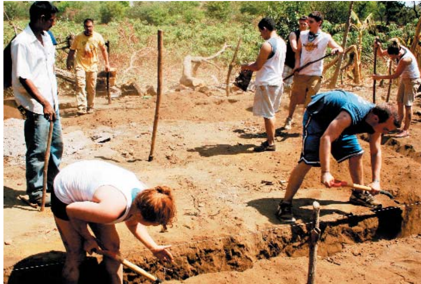
Students from the University of Birmingham dig footers for new houses.
